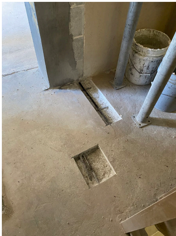
Picture 1: North stairwell repairs
