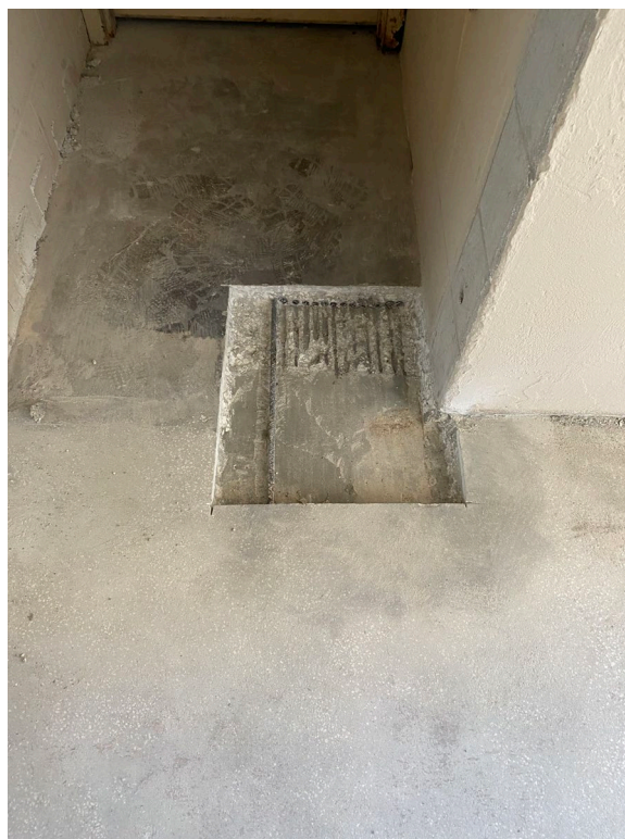
Picture 2: 3 rd floor trash room repair
